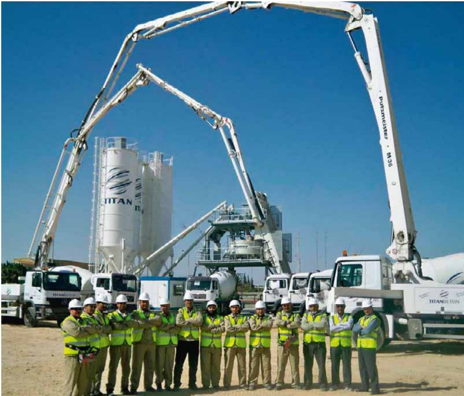
Safety training in ready-mix concrete plant, Alexandria, Egypt, 2009
