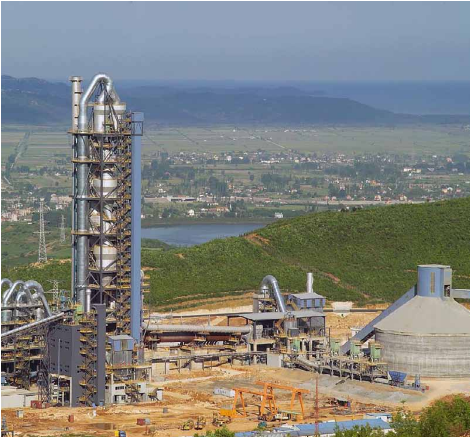
TITAN new cement plant in Albania
